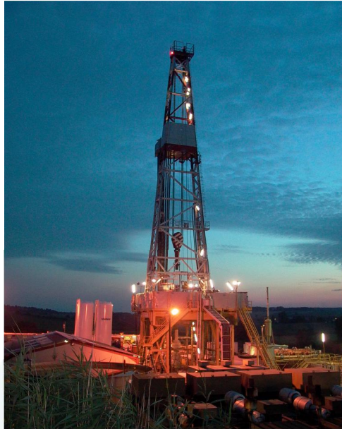
Rig installation in Soultz, France Hot Dry Rock project
