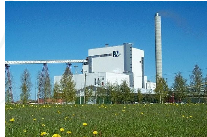
Alholmens Kraft, Finland Combustion power plant, 240 MWe
