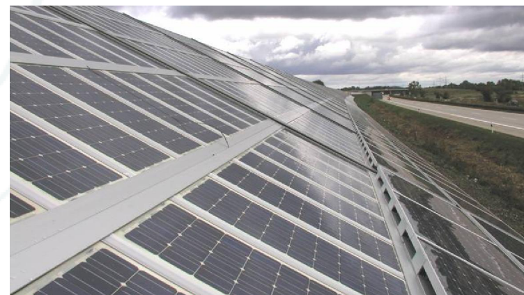
1.2 km sound barrier, A92 motorway, Germany
