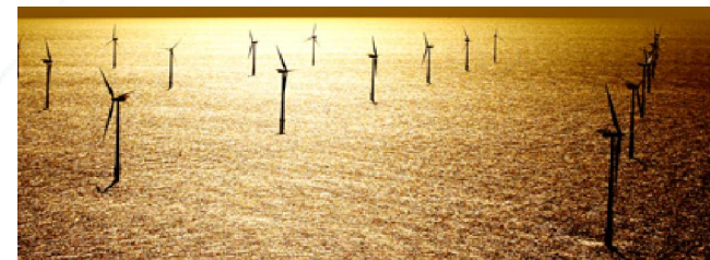
Horn Rev, Denmark, 160 MW
