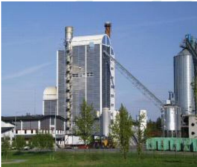
Värnamo, Sweden Integrated Gasification Combined Cycle, 6 MWe, 9MWth. CHRISGAS project
